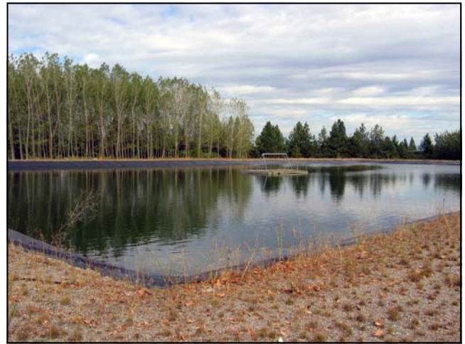
Lagoon Wastewater System
