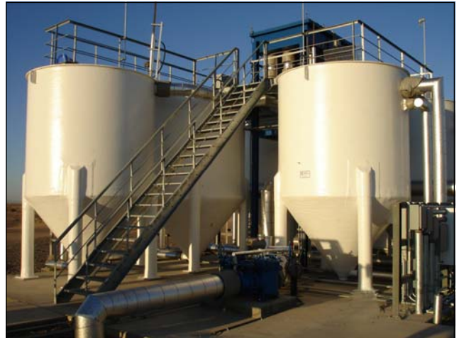
Featuring Centra-flo ™ continuous backwash sand filters.
