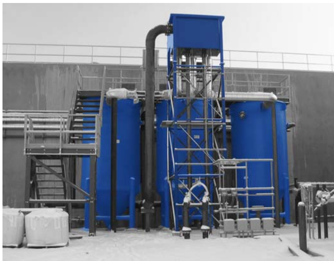
0.75 MGD (33 L/s) Centra-flo™ installation in New York
